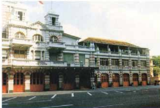
▼ Central Fire Station at Hill Street.
